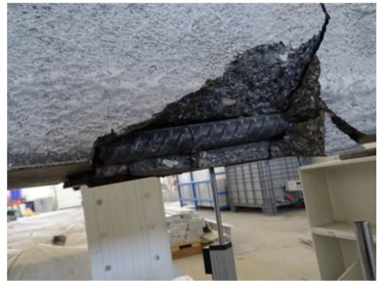
Fig. 2 The beam specimen with no fiber after failure
